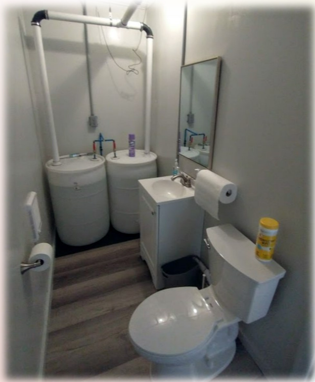
The Newly Renovated and Remodeled Bathroom
